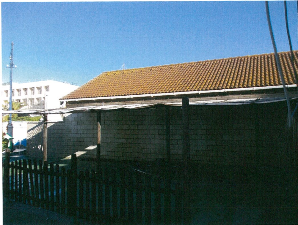
Fig 8 Timber lean too structure against sea scouts building
