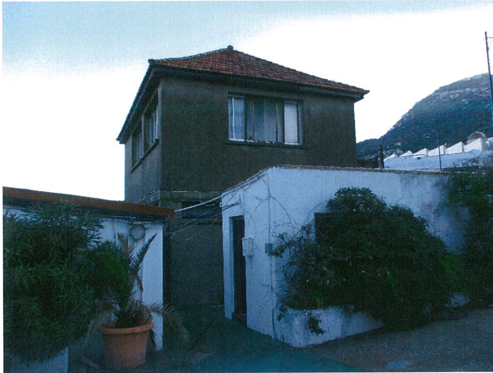
Fig 1 Two storey structure
