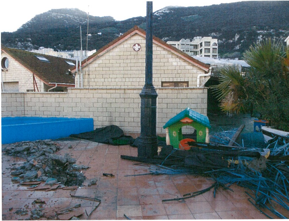
Fig 7 Boundary wall with sea scouts property
